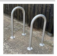
The tubular cycle stand, a familiar sight throughout the UK, allows the frame of the bicycle to be secured by the users own security lock.
